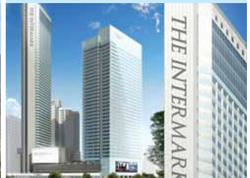
The Intermark Tower, Malaysia
