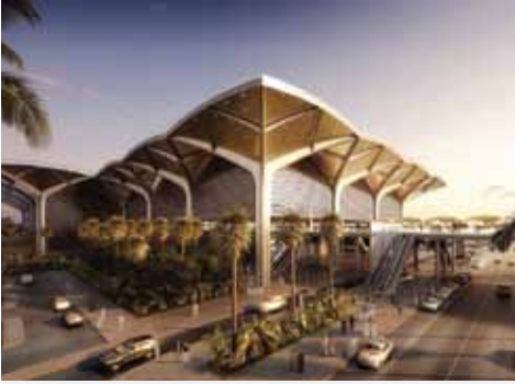
Harmain Railways, KSA
